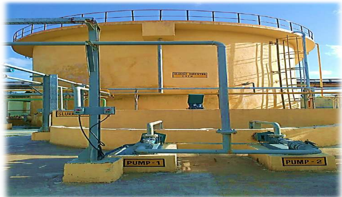
Actual site picture of Anaerobic Digester at Dinshaw's Nagpur
